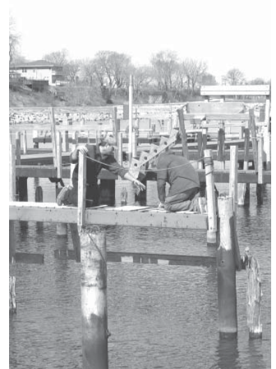
Mike Dziubek and Ted Ingrassia remove decking at the April 4 Slip and Waterfront Work Party.
